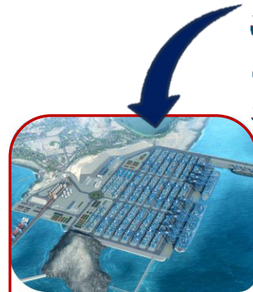
Chancay Port Terminal Scheduled to begin operations in November 2024.
